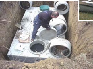
Replacing a septic tank and drain field
