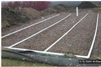
Replacing a septic tank and drain field
